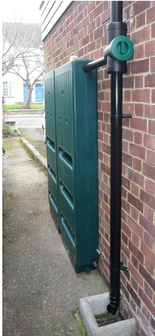
Ultra Slim Wall Tank System 470 litres can replace 20% of your potable water used for toilet flushing
